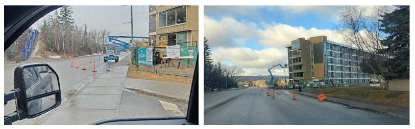
The sidewalk closed signage is placed outside of the sightline from the nearest marked crosswalk on Dominion.
