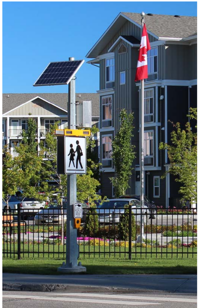
Figure 3: Rapid Rectangular Flashing Beacon (RRFB) – 20th Avenue at Oak Street
