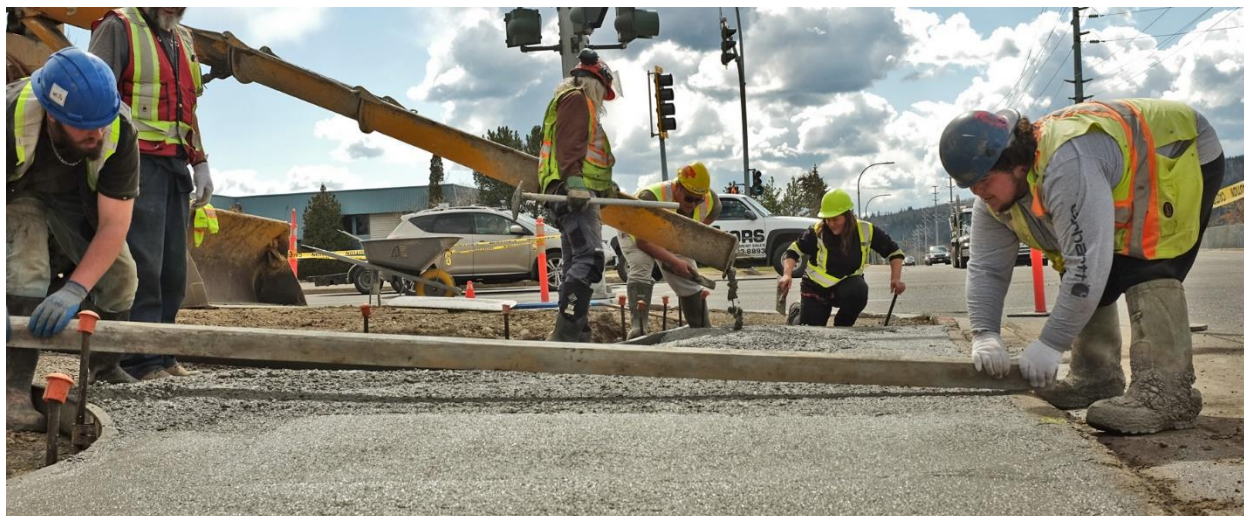
Building sidewalks. Source: City of Prince George
