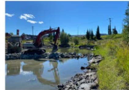
Crews working to renew a pond
