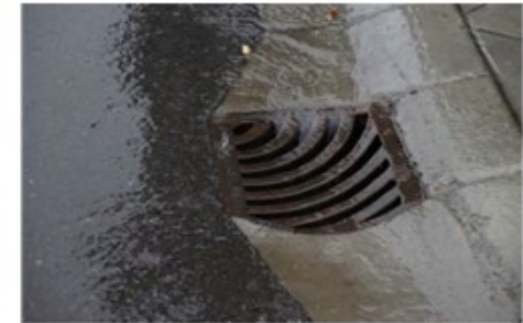
Renewed catch basin
