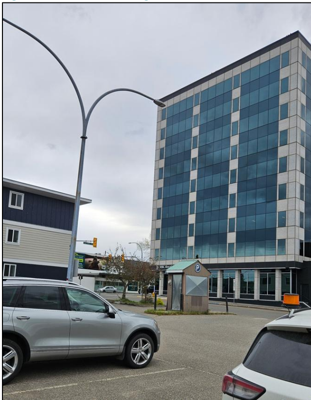
Figure 6-24: RBC Building Near P4 Earl Brown Lot
