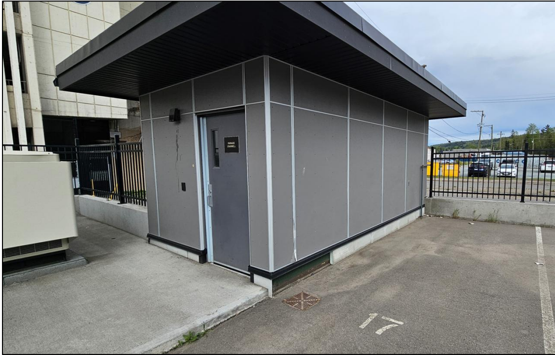
Figure 6-2: P10 George Street Parkade Stairwell Shelter
