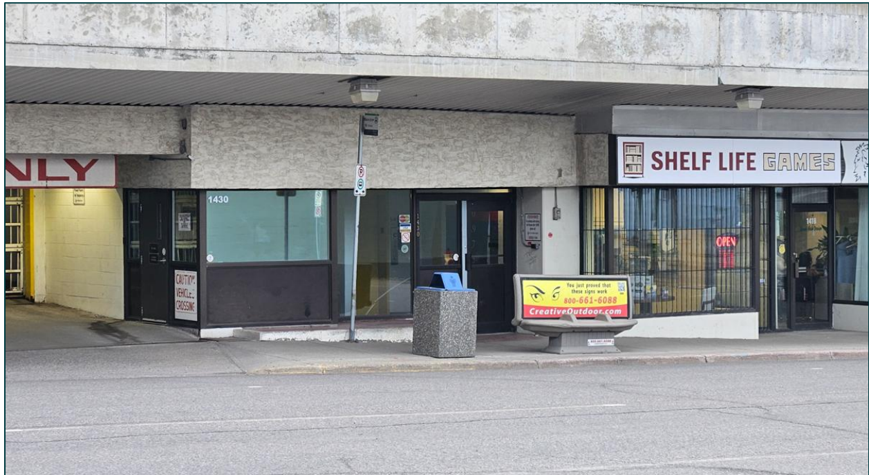
Figure 6-15: Lack of Signage Outside of P9 2 nd Ave Parkade
