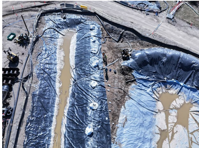
Project runoff water is collected in holding ponds onsite.
