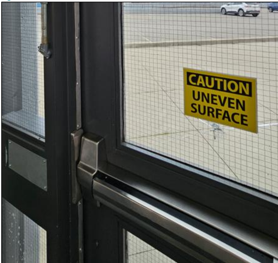
Figure 6-19: Cracked Window at Ground Level Door
