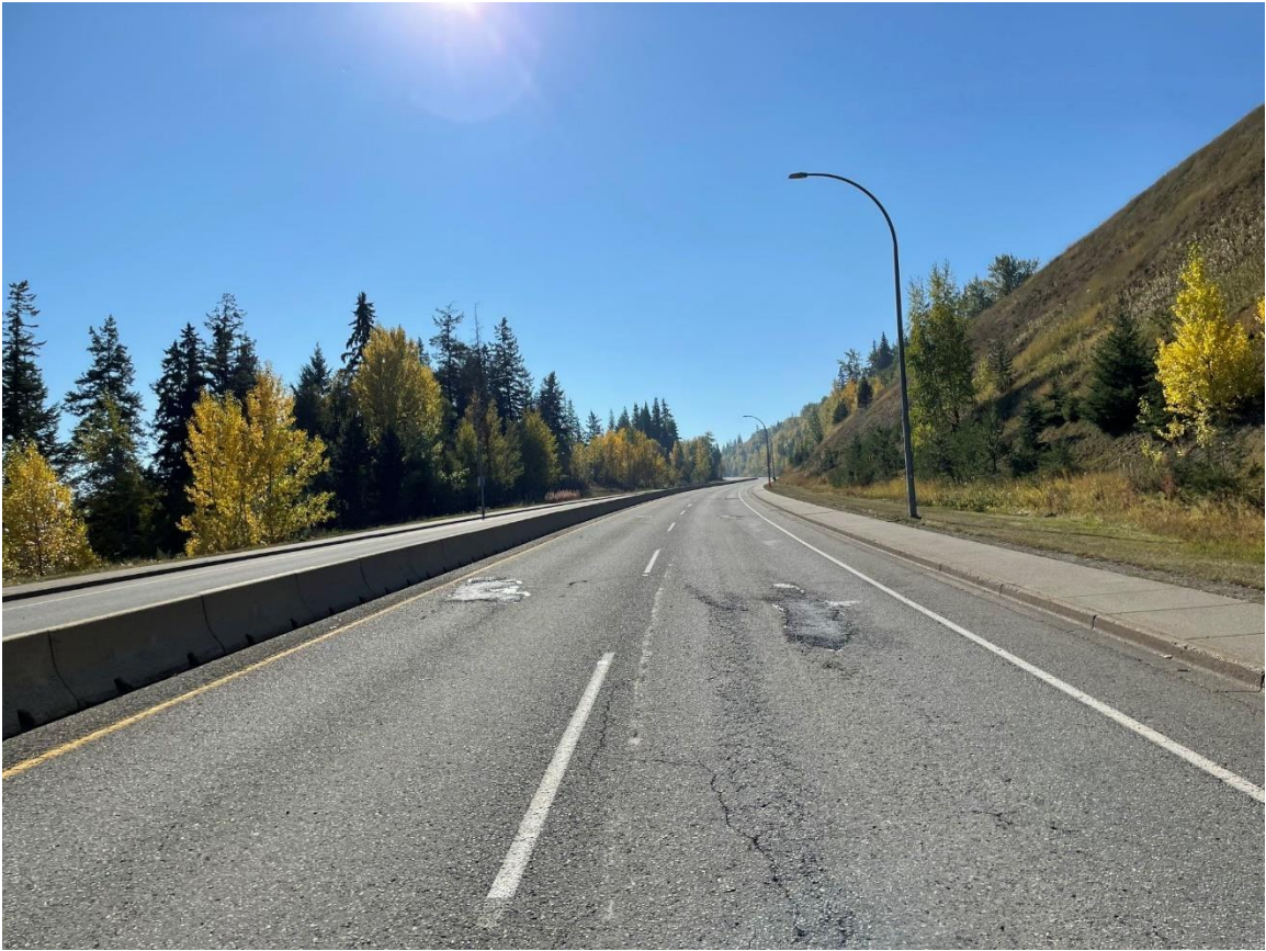
University Way– looking south, before road rehabilitation.
