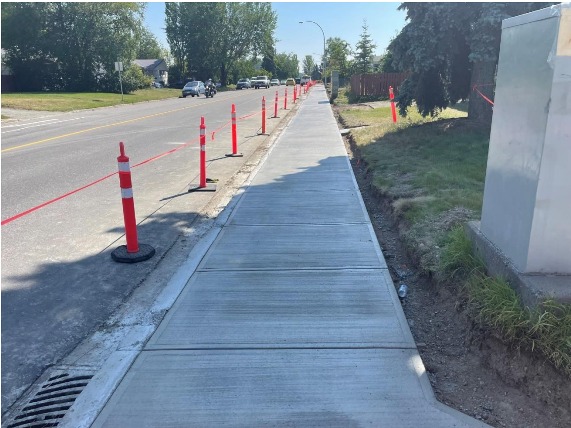
Carney Street Sidewalk - looking south near 15 th Avenue, after sidewalk rehabilitation.
