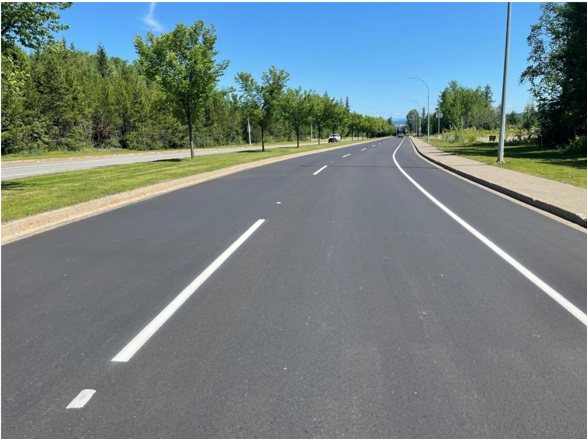
Ospika Boulevard - looking north near Tyner Boulevard, after road rehabilitation.
