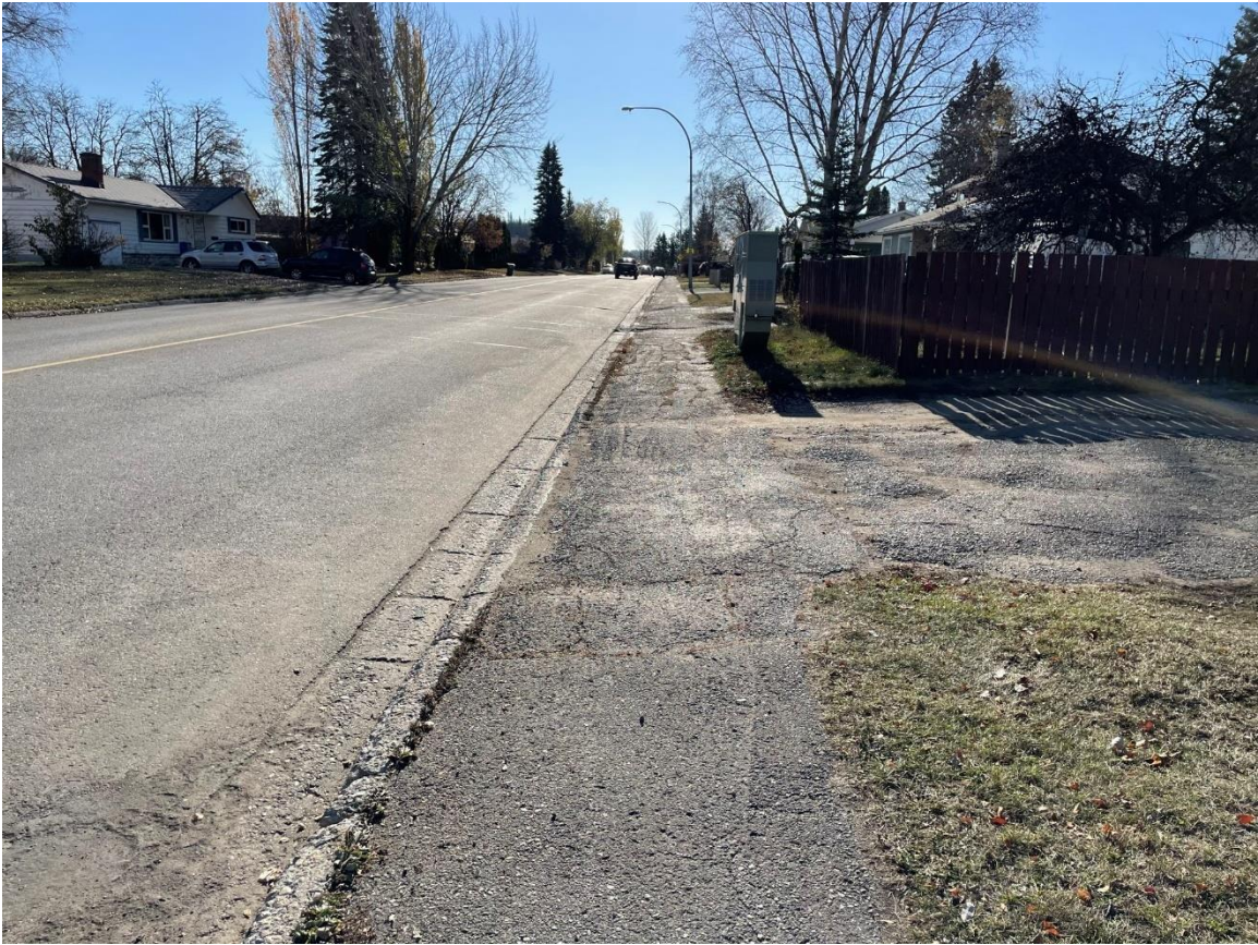
Carney Street Sidewalk - looking south near 15 th Avenue, before sidewalk rehabilitation.
