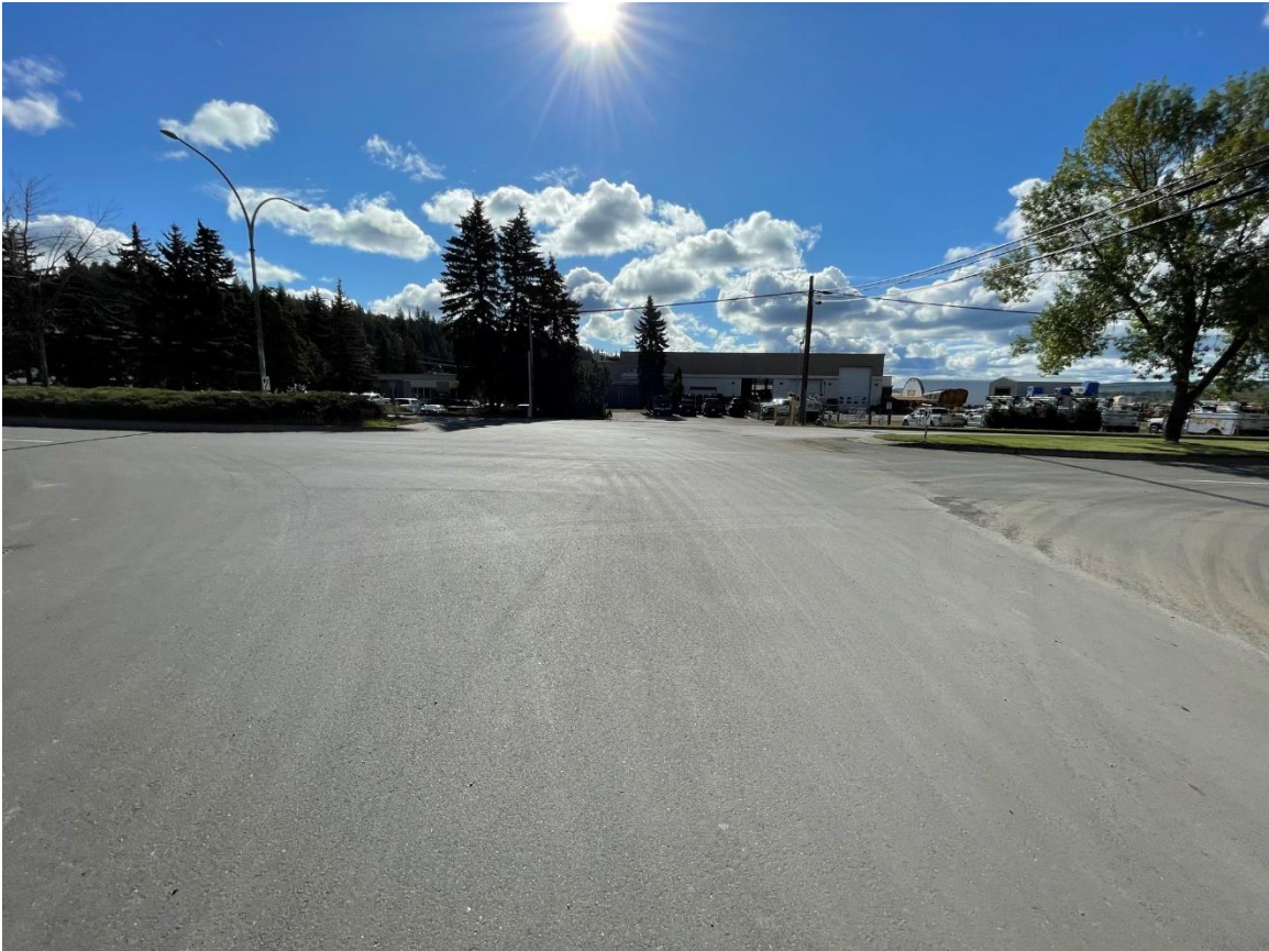
Great Street – looking south towards Terminal Boulevard, after road rehabilitation.
