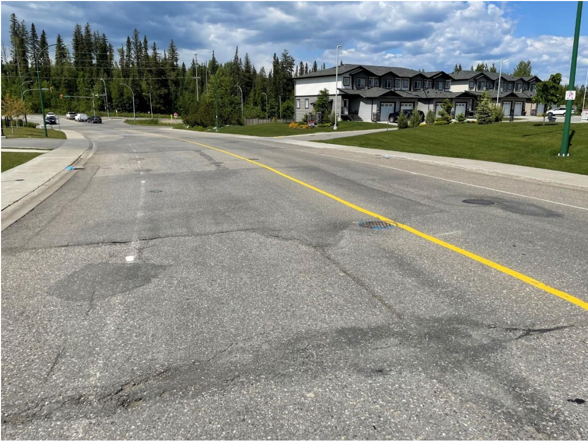
Westgate Avenue - looking north near Cathedral Avenue, before road rehabilitation.
