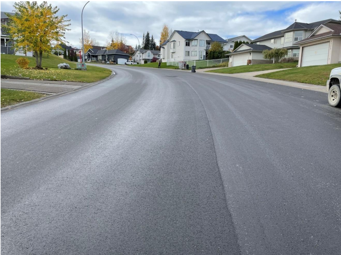
St Lawrence Avenue - looking west near Southridge Avenue, after road rehabilitation.
