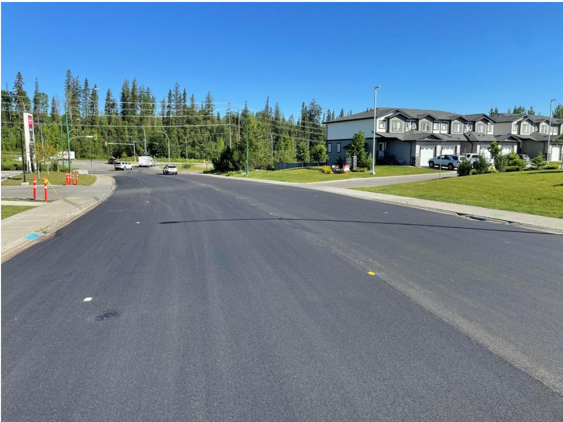
Westgate Avenue - looking north near Cathedral Avenue, after road rehabilitation.
