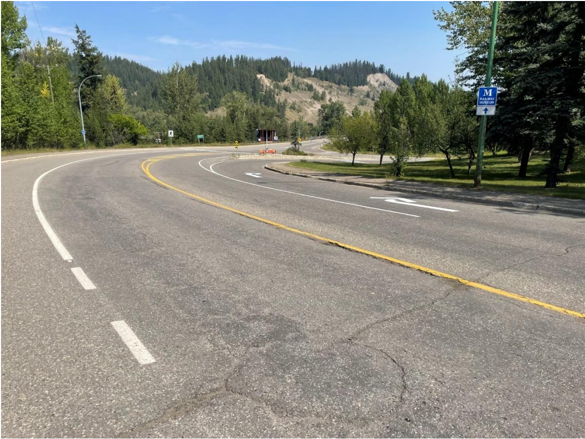
Carney Street – looking northeast towards 1 st Avenue, before road rehabilitation.
