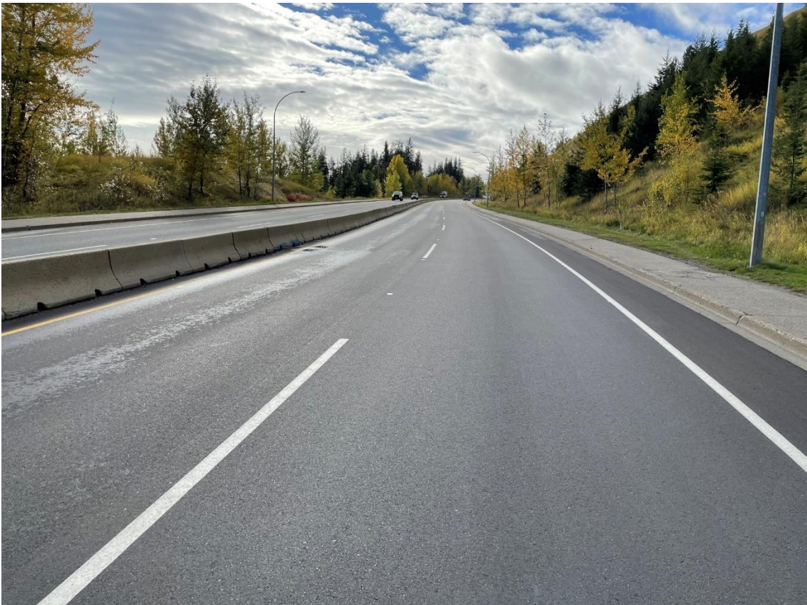
University Way– looking south, after road rehabilitation.
