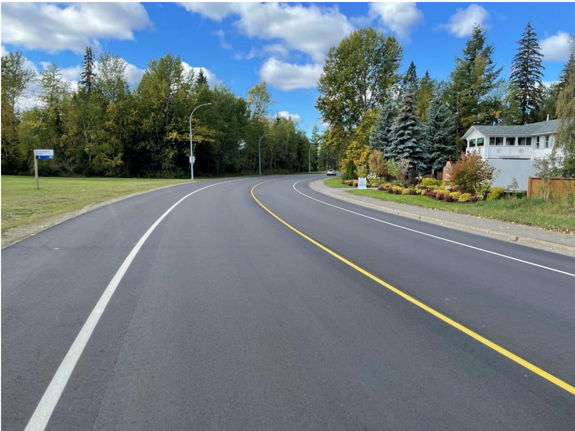
Ferry Avenue – looking southwest near Clapperton Street, after road rehabilitation.
