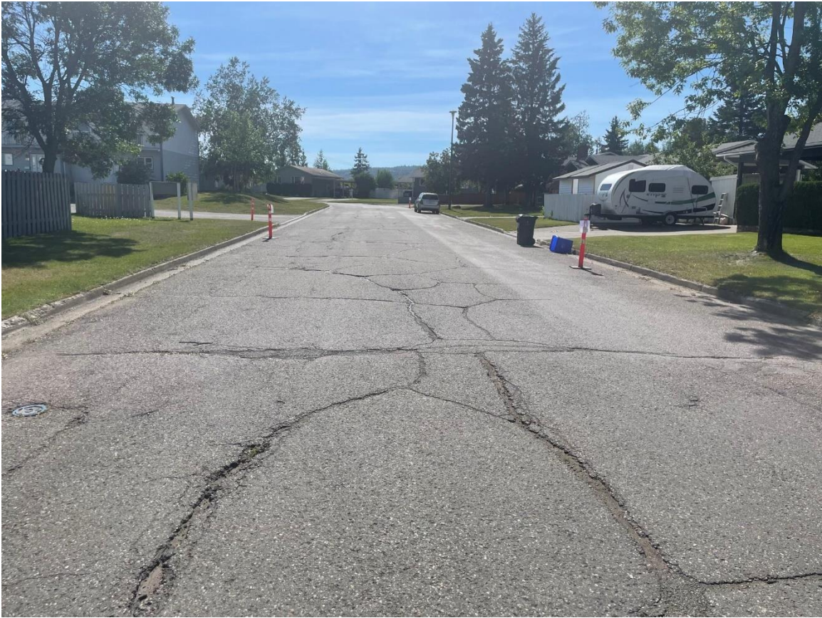
Boyd Street – looking south near Clark Crescent, before road rehabilitation.
