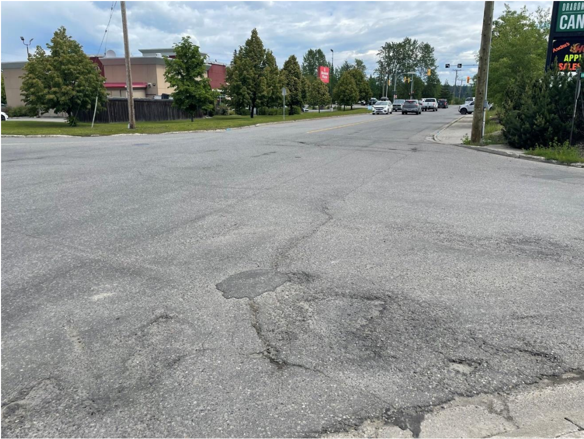
Vance Road - looking east from Hollandia Drive, before road rehabilitation.
