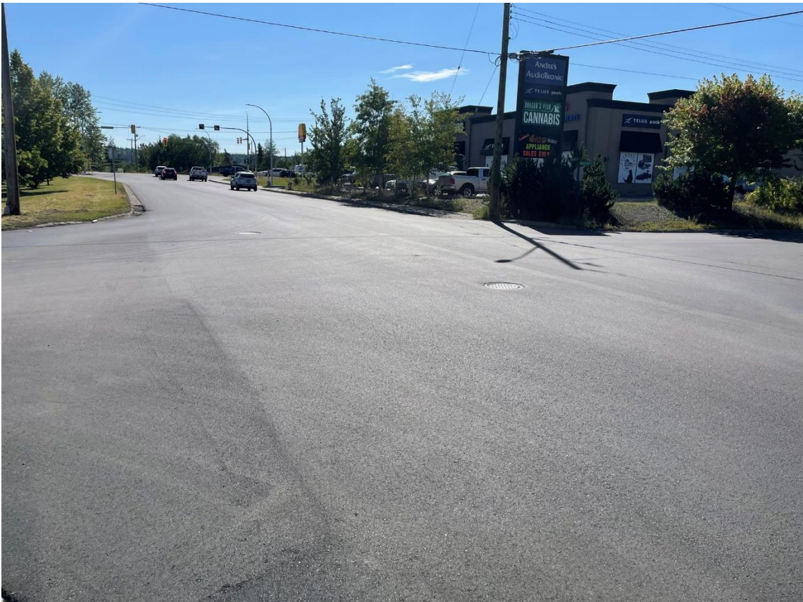
Vance Road - looking east from Hollandia Drive, after road rehabilitation.
