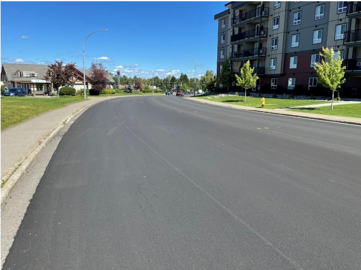
Dakelh Ti - looking north near Stringer Crescent, after road rehabilitation.
