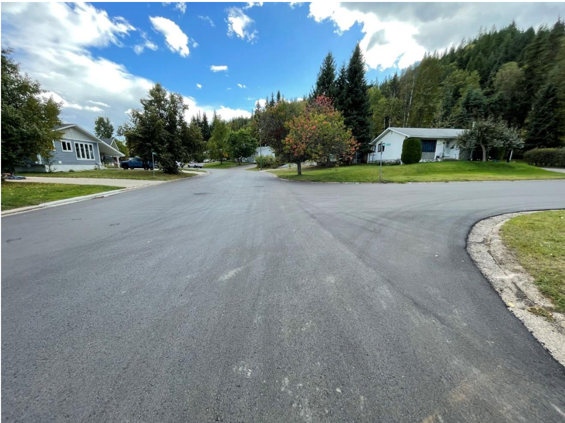
Webber Crescent – Looking south towards Rush Place, after road rehabilitation.
