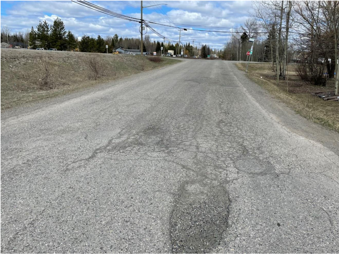
Hart Highway Frontage – looking north towards Estavilla Drive, before road rehabilitation.
