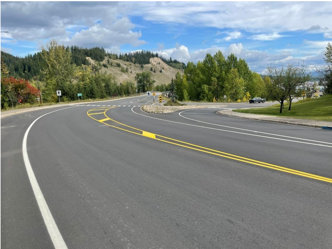
Carney Street – looking northeast towards 1 st Avenue, after road rehabilitation.
