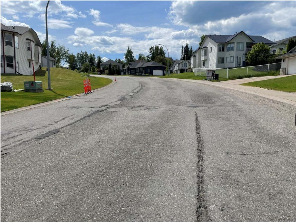
St Lawrence Avenue - looking west near Southridge Avenue, before road rehabilitation.
