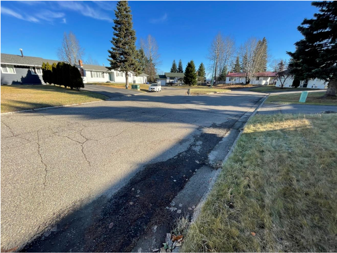
Quesnel Avenue – looking east, before road rehabilitation.
