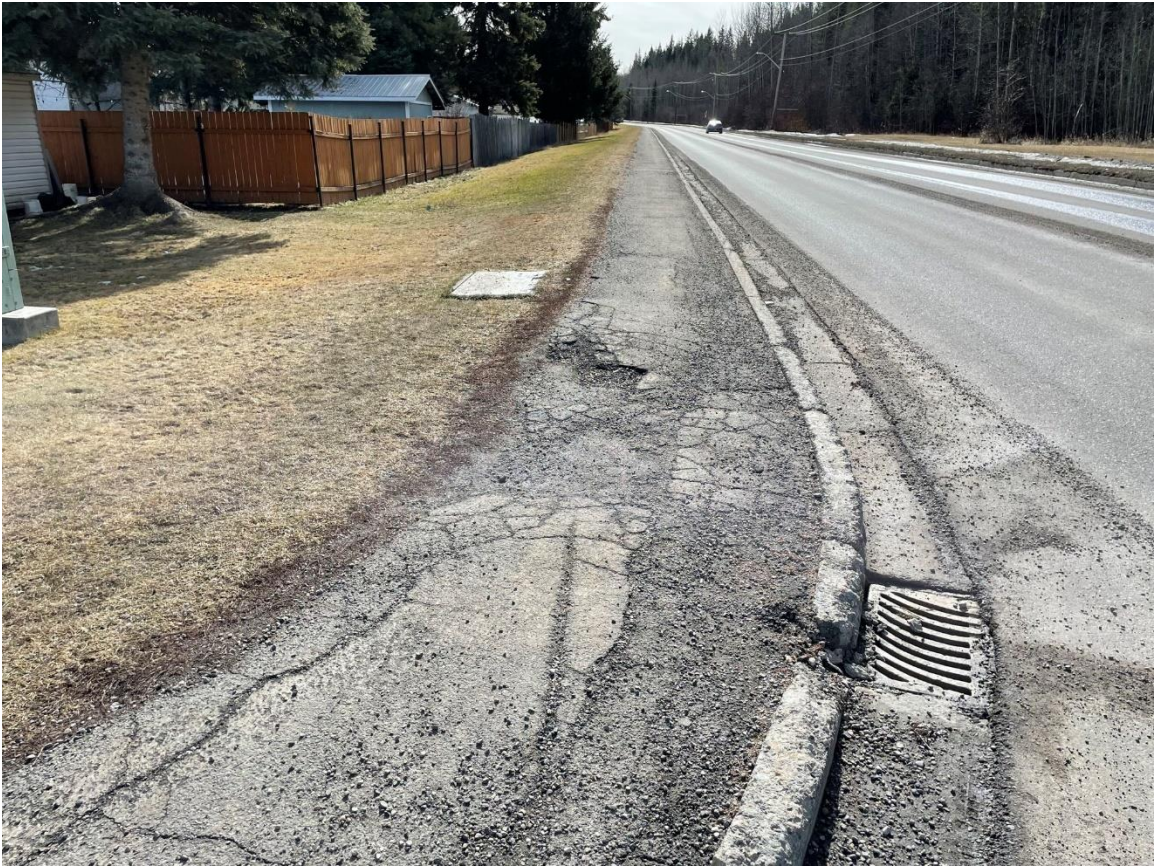
Domano Boulevard Sidewalk – Looking south from Gladstone Drive, before asphalt sidewalk rehabilitation.
