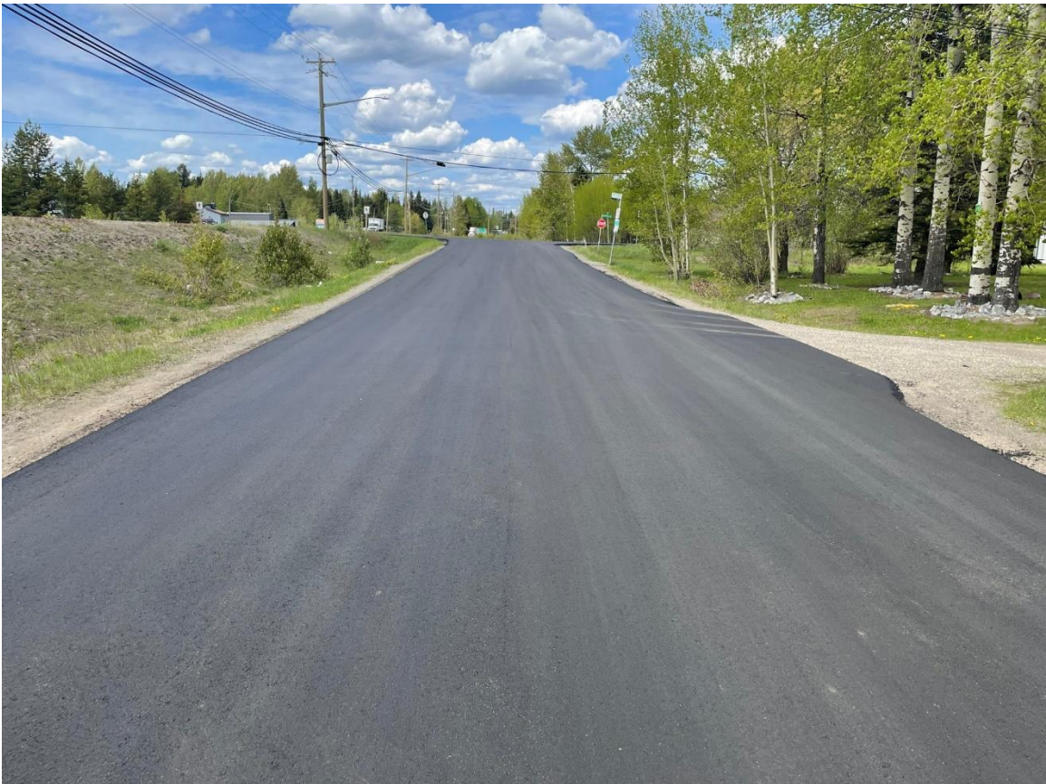
Hart Highway Frontage – looking north towards Estavilla Drive, after road rehabilitation.
