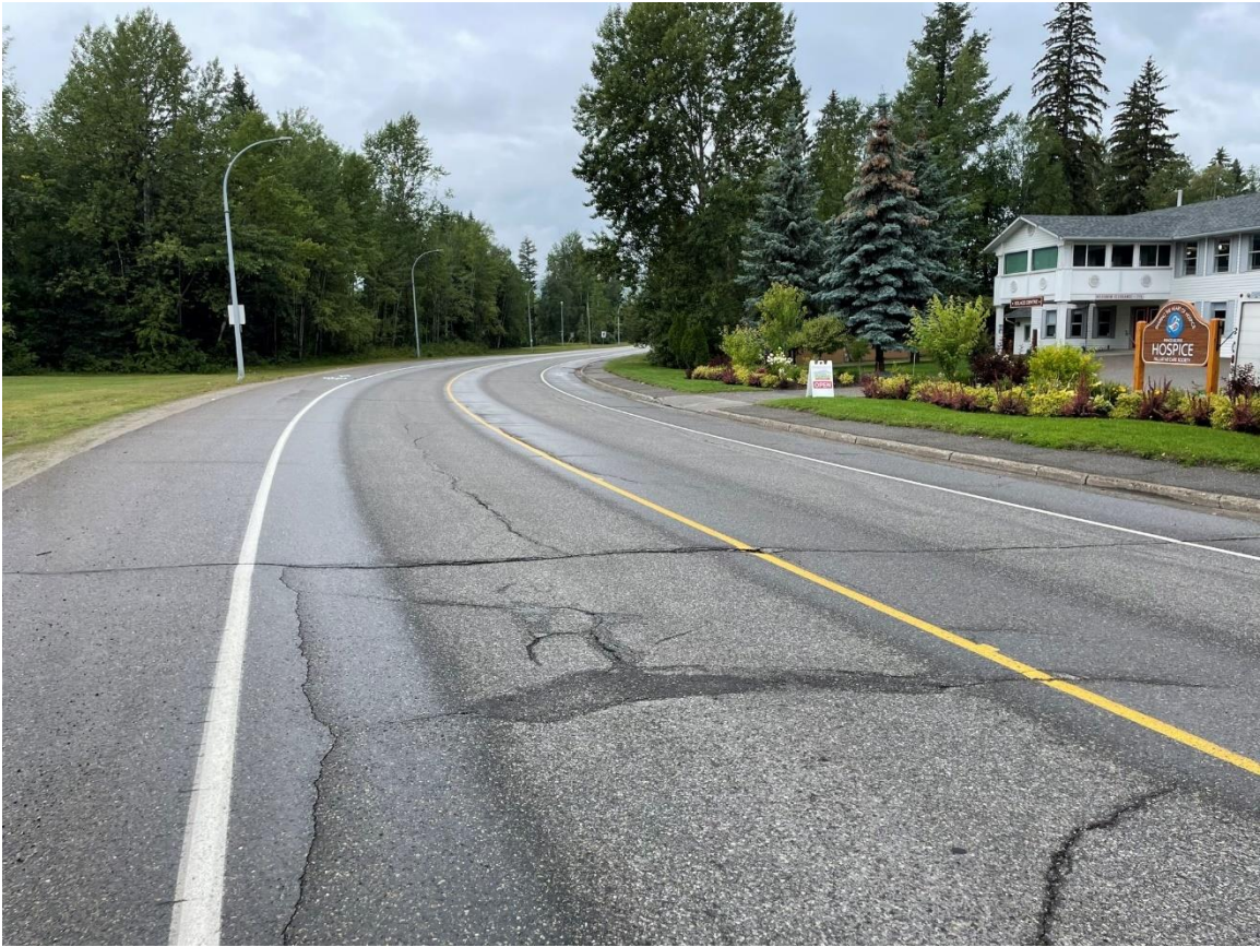
Ferry Avenue – looking southwest near Clapperton Street, before road rehabilitation.
