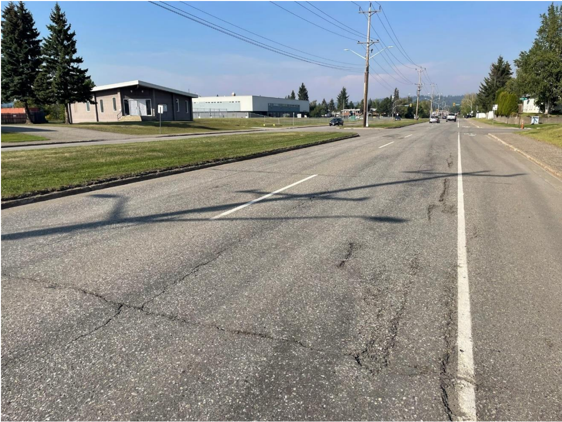
Ospika Boulevard – looking north near Parsnip Crescent, before road rehabilitation.
