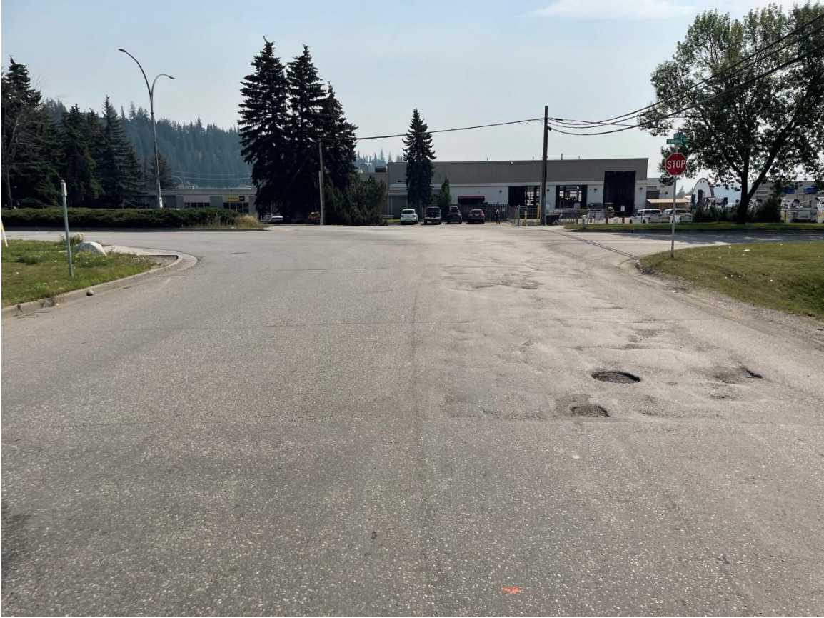
Great Street – looking south towards Terminal Boulevard, before road rehabilitation.
