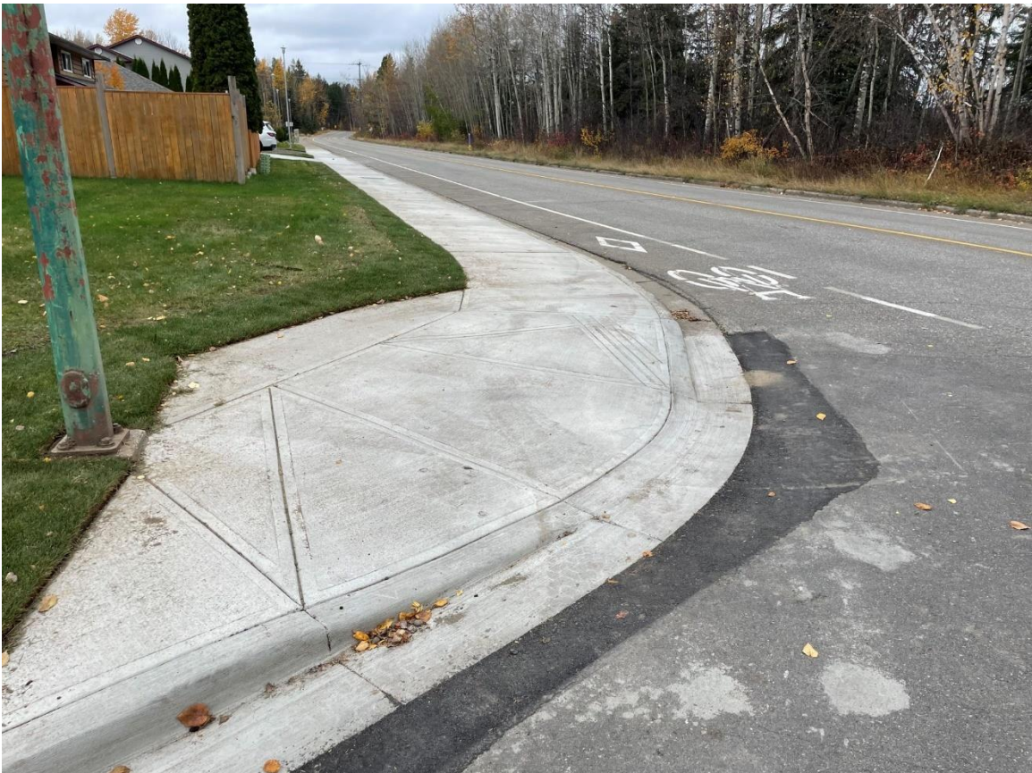
Ospika Boulevard Sidewalk – Looking west from McGowan Drive, before new sidewalk installation.
