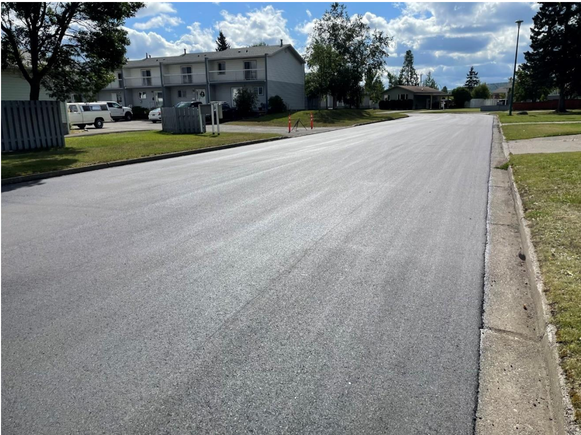
Boyd Street – looking south near Clark Crescent, after road rehabilitation.
