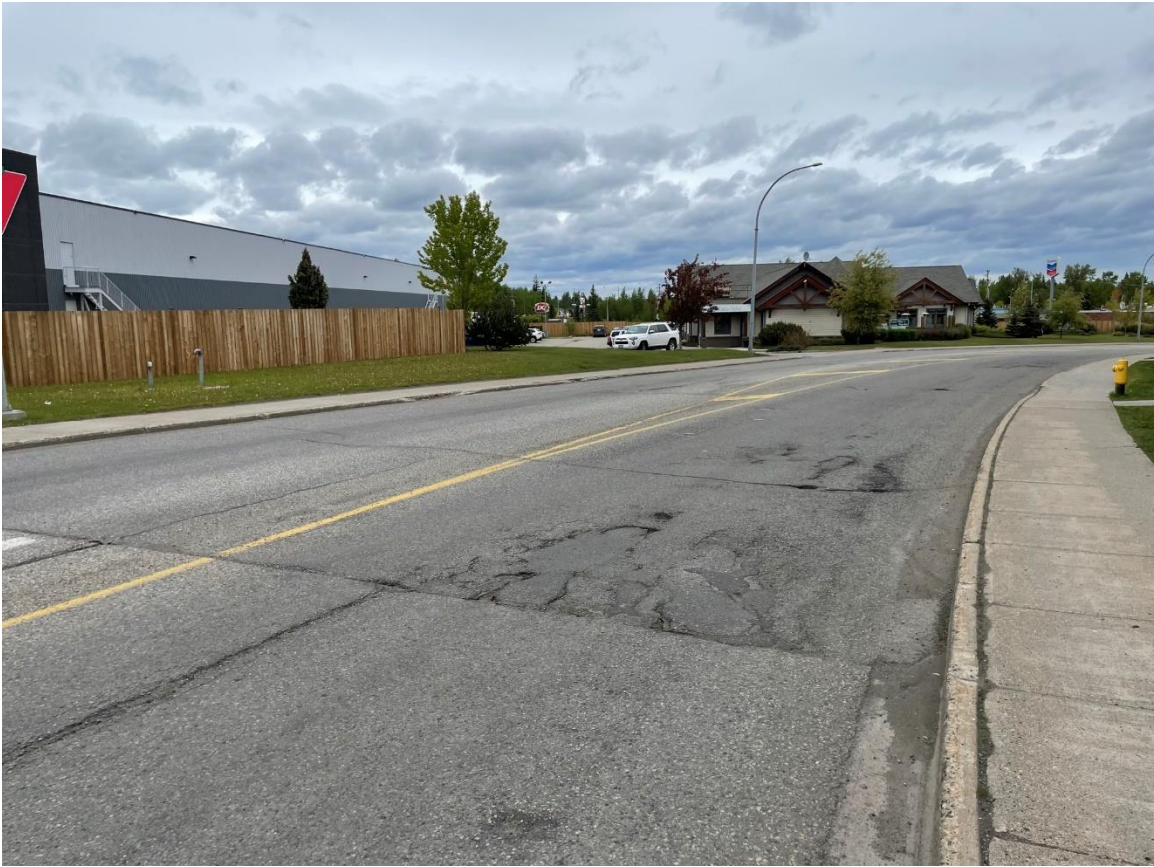
Dakelh Ti - looking north near Stringer Crescent, before road rehabilitation.
