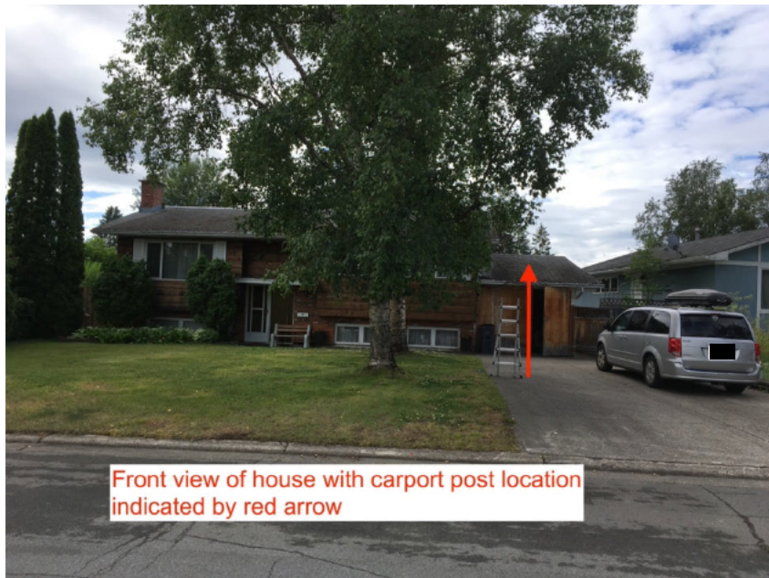
Figure 5: Front view of house from neighbor across the street. Red arrow / ladder indicates carport post position distance from the road.
