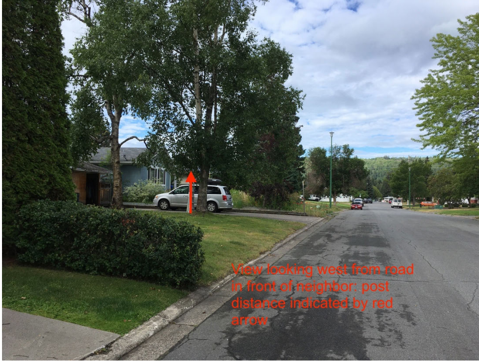
Figure 1: View looking along the street toward the west. The red arrow indicates the proposed distance of the carport posts.
