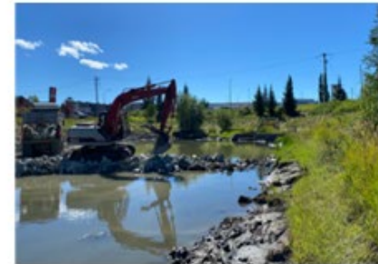
Crews working to renew a pond
