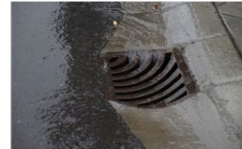
Renewed catch basin
