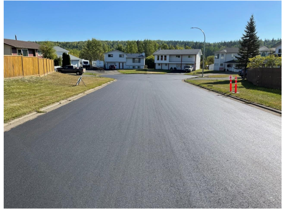
Moledo Place – looking east near Bittner Road West, after road rehabilitation. The curb island was removed, and streetlight relocated to the boulevard.
