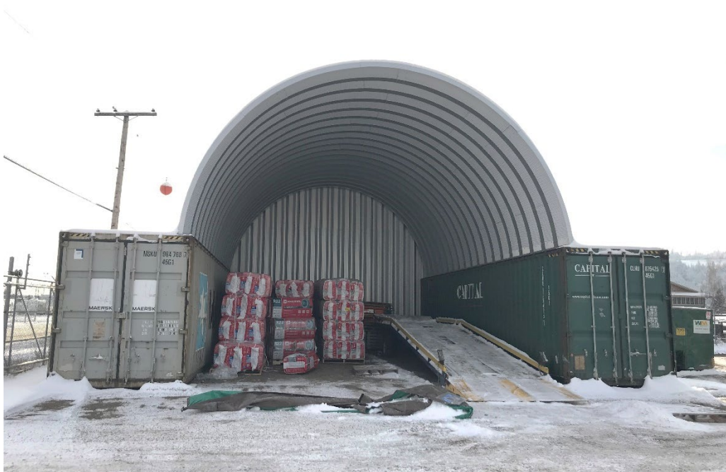
From the subject property, south facing the existing accessory building.
