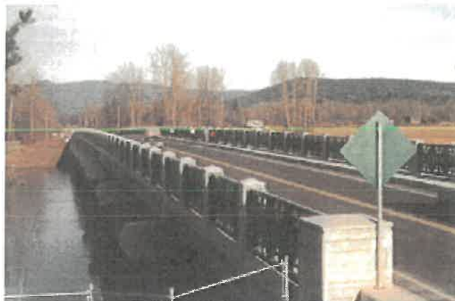
Jacob Haldi Bridge, Fort Langley BC
