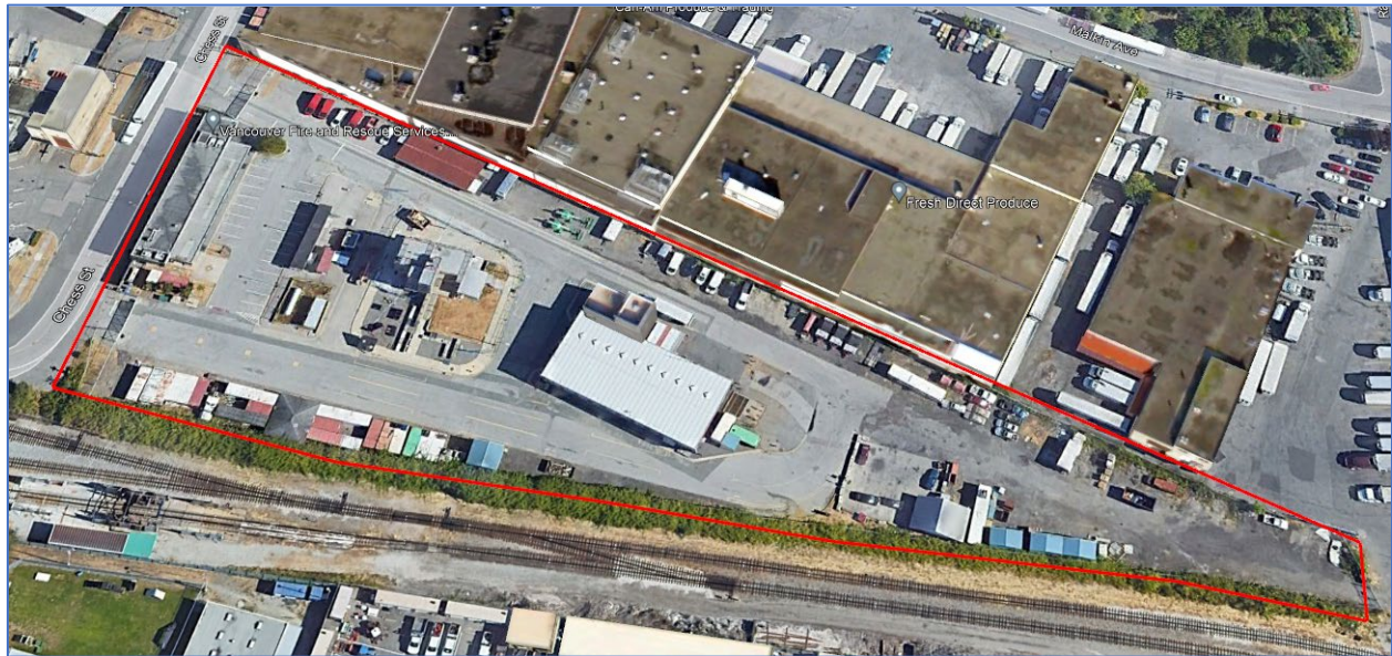
Figure 32: Vancouver Fire Training Site at Chess Street, approximately 11,600 square metres.
