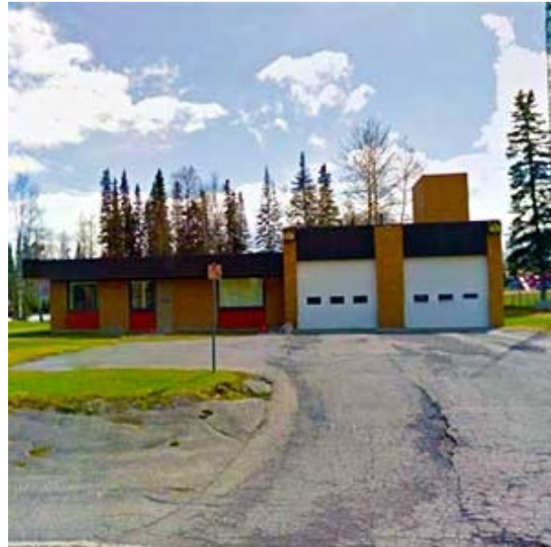
Figure 31: Hall 4 - 6555 Kelly Road South
