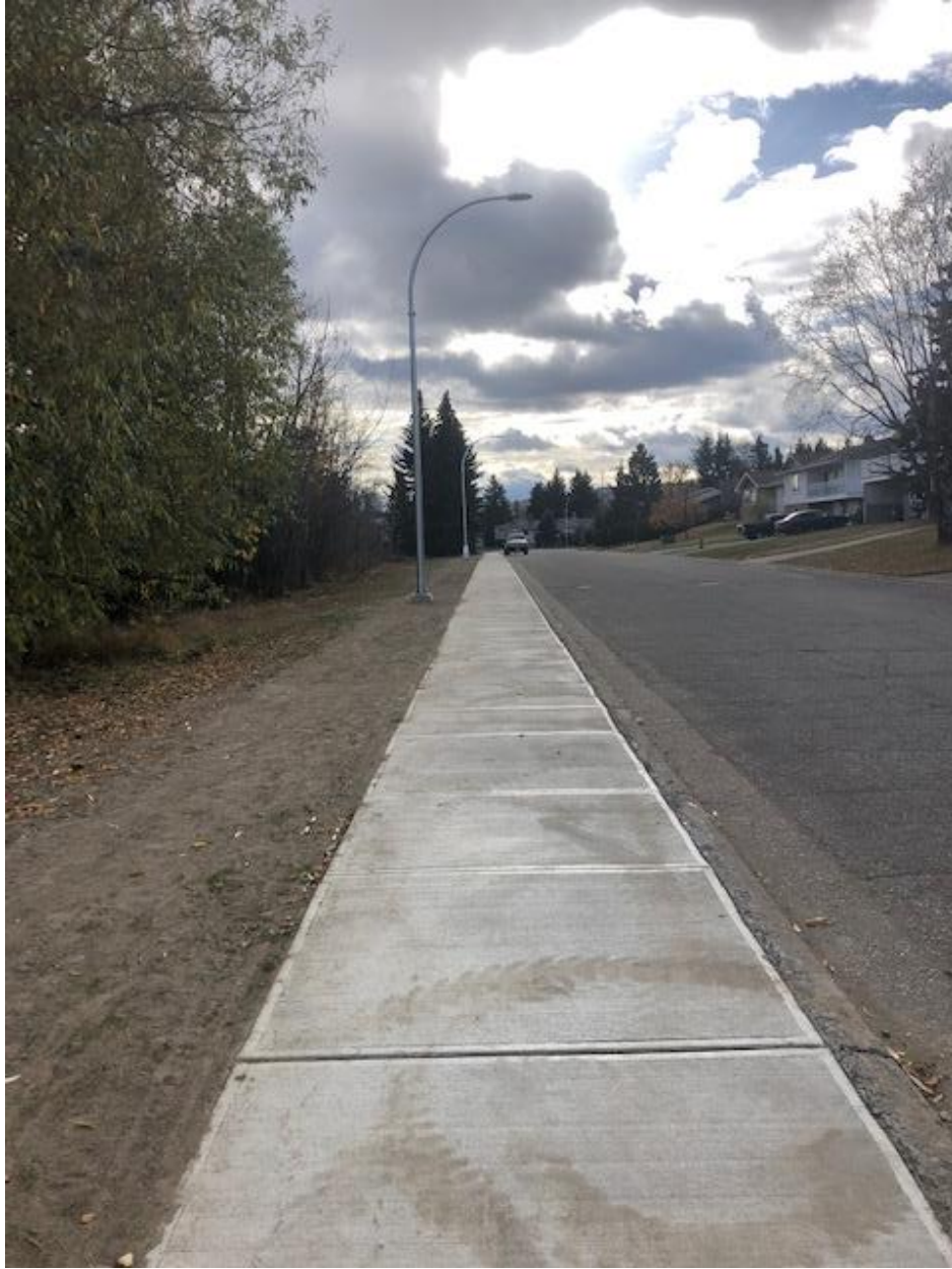
New sidewalk Kerry St between Ospika and Rainbow looking south after. Six new streetlights installed on a single feed with control panel. The three previous streetlights all had single feeds direct from Hydro vaults.
