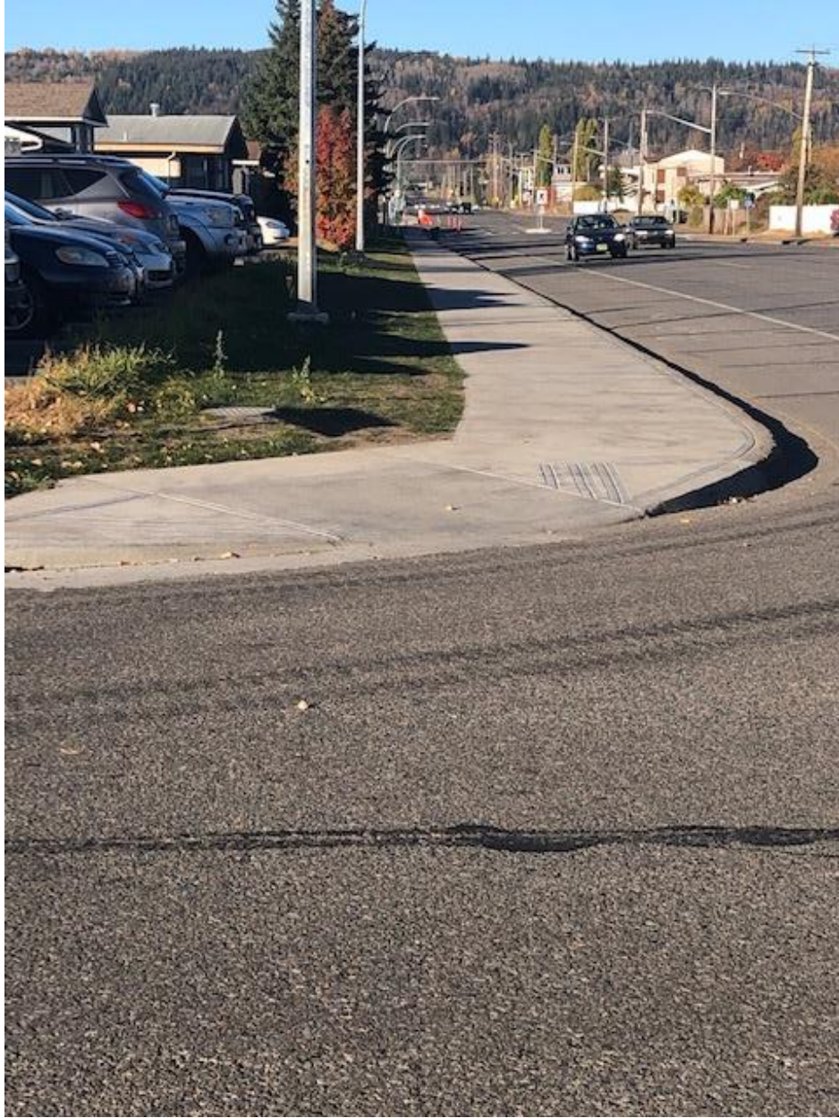
5 th and Union after renewal. Typical accessibility letdown. 42 letdowns will be completed in 2022.
