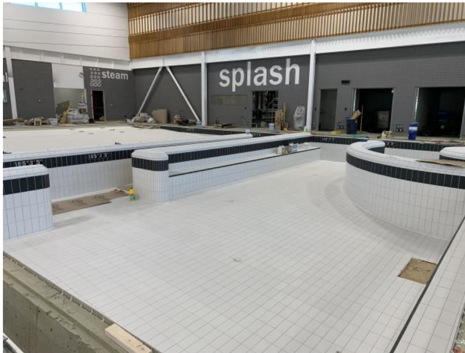
Leisure pool and wave pool tile work.
