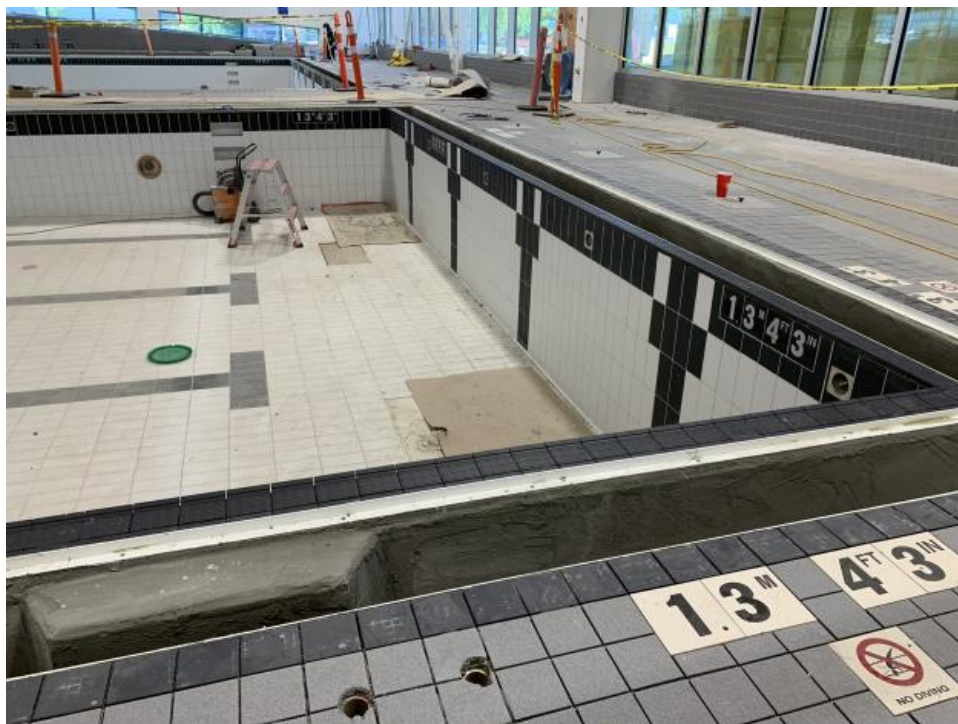
Teach pool tile with depth markers under construction.
