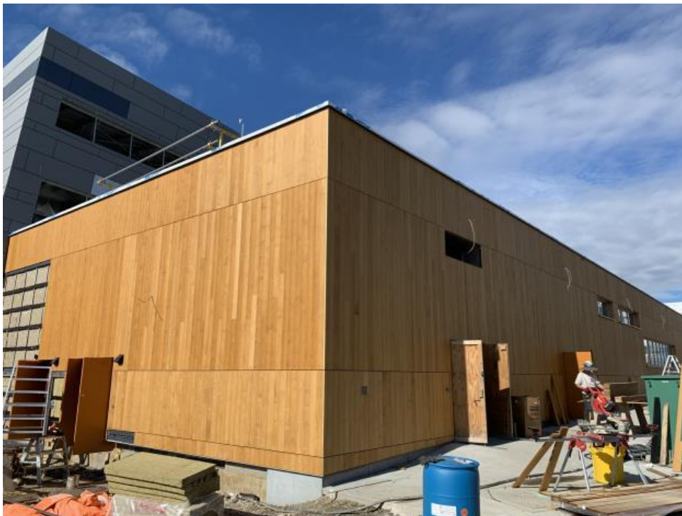
Accoya wood siding at the northeast corner by Dominion Street.
