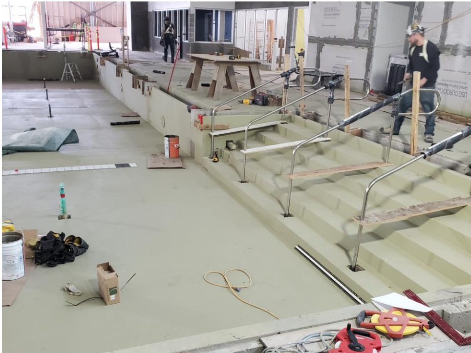
Teach pool tank staircase entrance.
