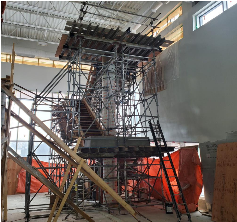
Waterslide tower under construction.
