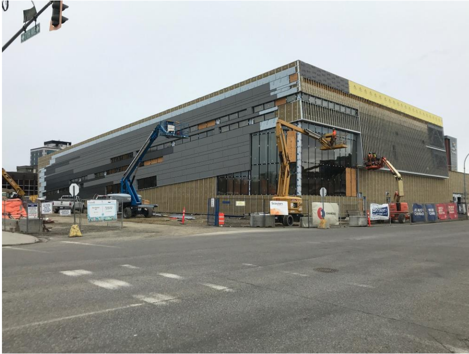
Exterior cladding installation underway at 7 th Avenue and Dominion Street.
